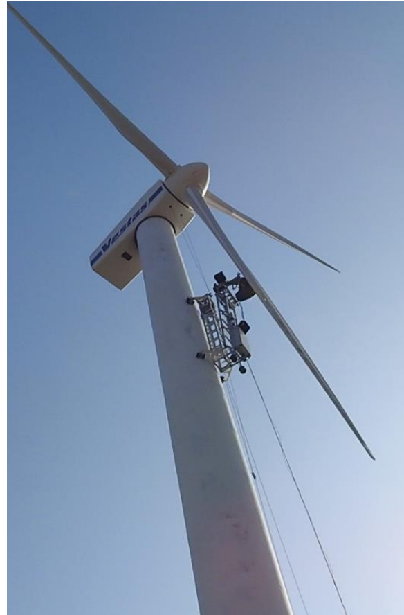
SheaRIOS inspection of in-situ a WTB
